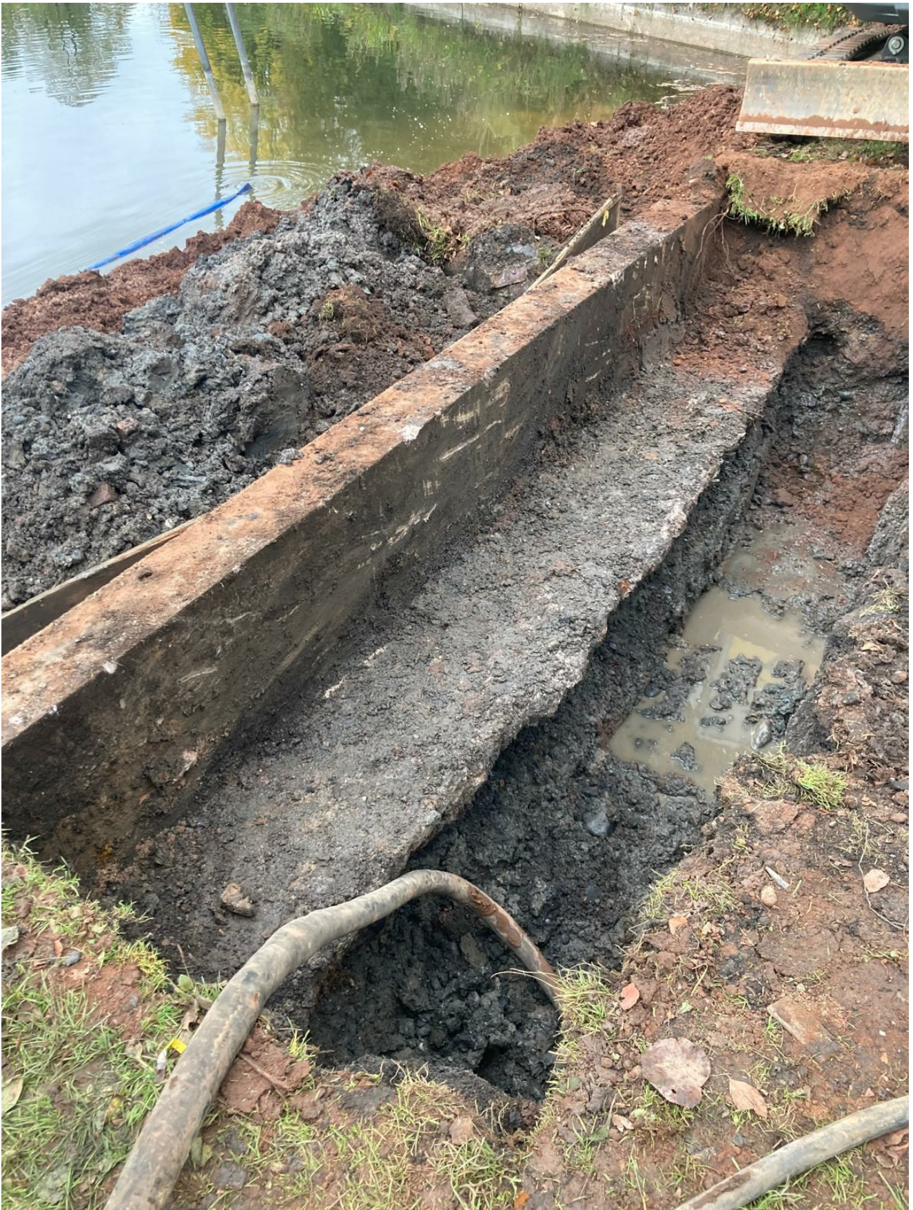
Photo showing excavated section of wall foundation and the void found
