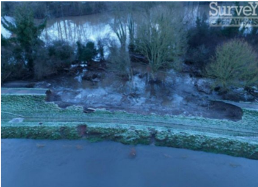
Photo of embankment breach
