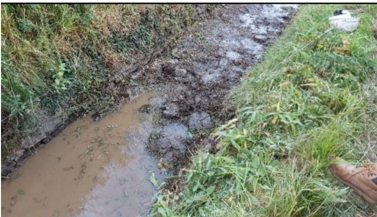
Photo 2: Earth that has built up in the spillway channel prior to cleaning.
