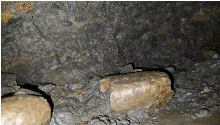
View above culvert crown looking downstream
